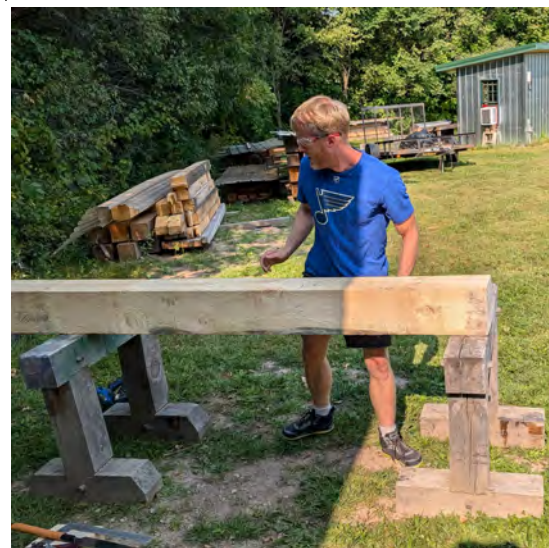
Sawhorses used to support work for layout
