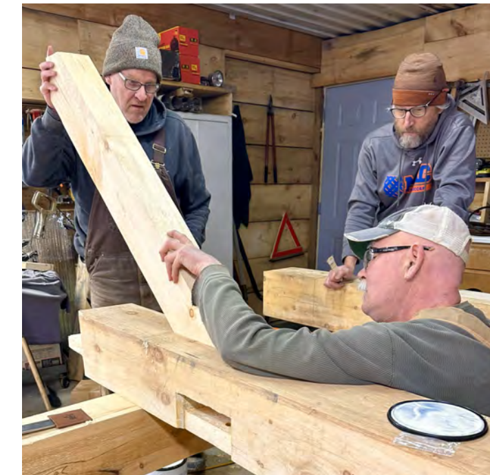
Checking a mortise pocket with a knee brace
