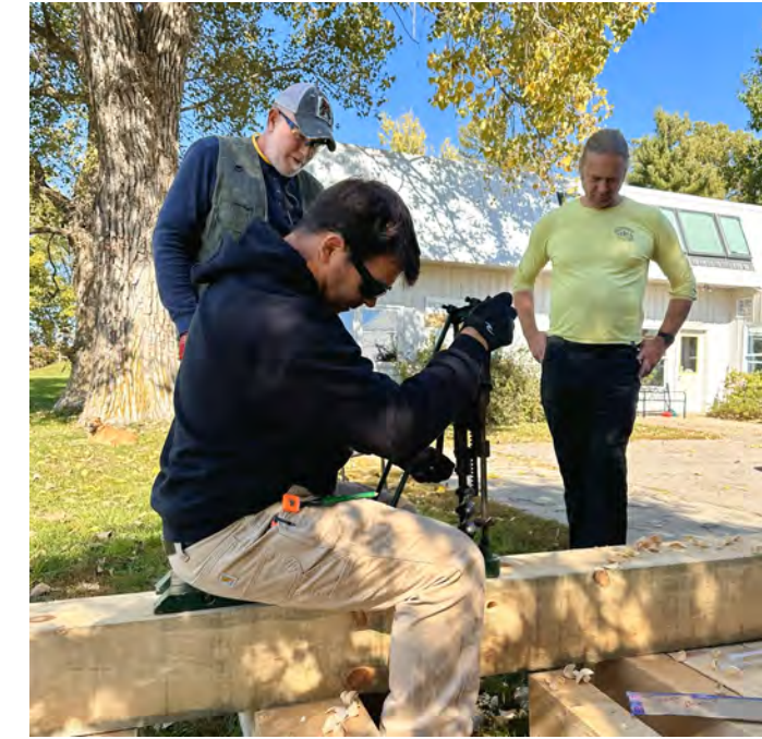
Cutting a mortise using a boring machine
