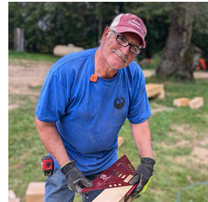
Knee brace layout with EZ Brace Revision 1 (4.8.25) Copyright 2025 - Star Hill Timberworks LLC
