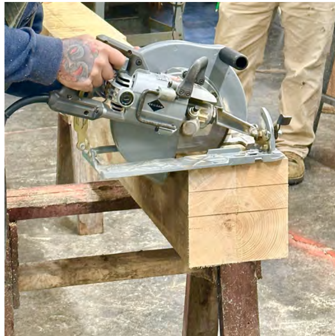
Cutting reference shoulder
