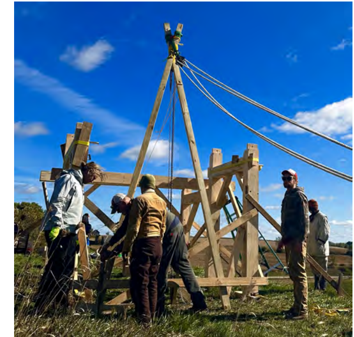
Raising sauna with a lifting shear
