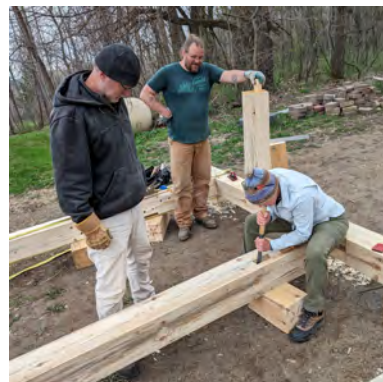
Test fitting a door header on a wall
