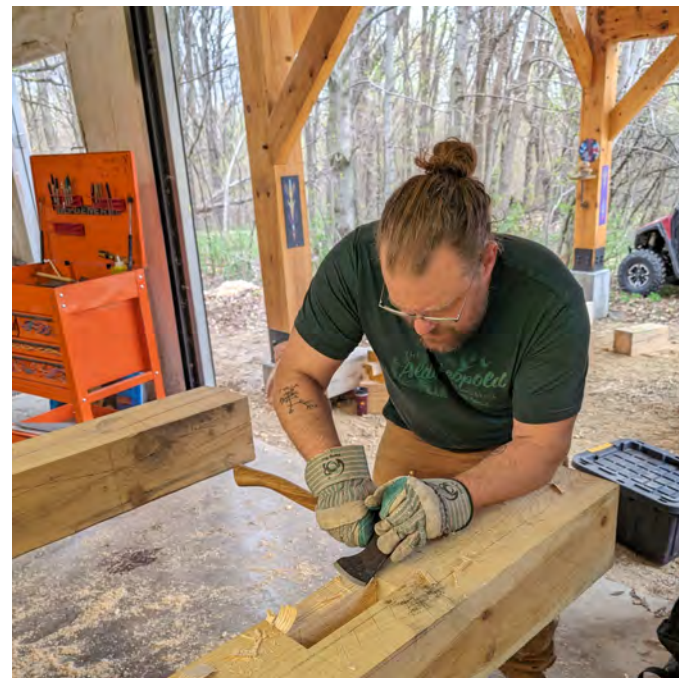
Cutting a housing with an axe
