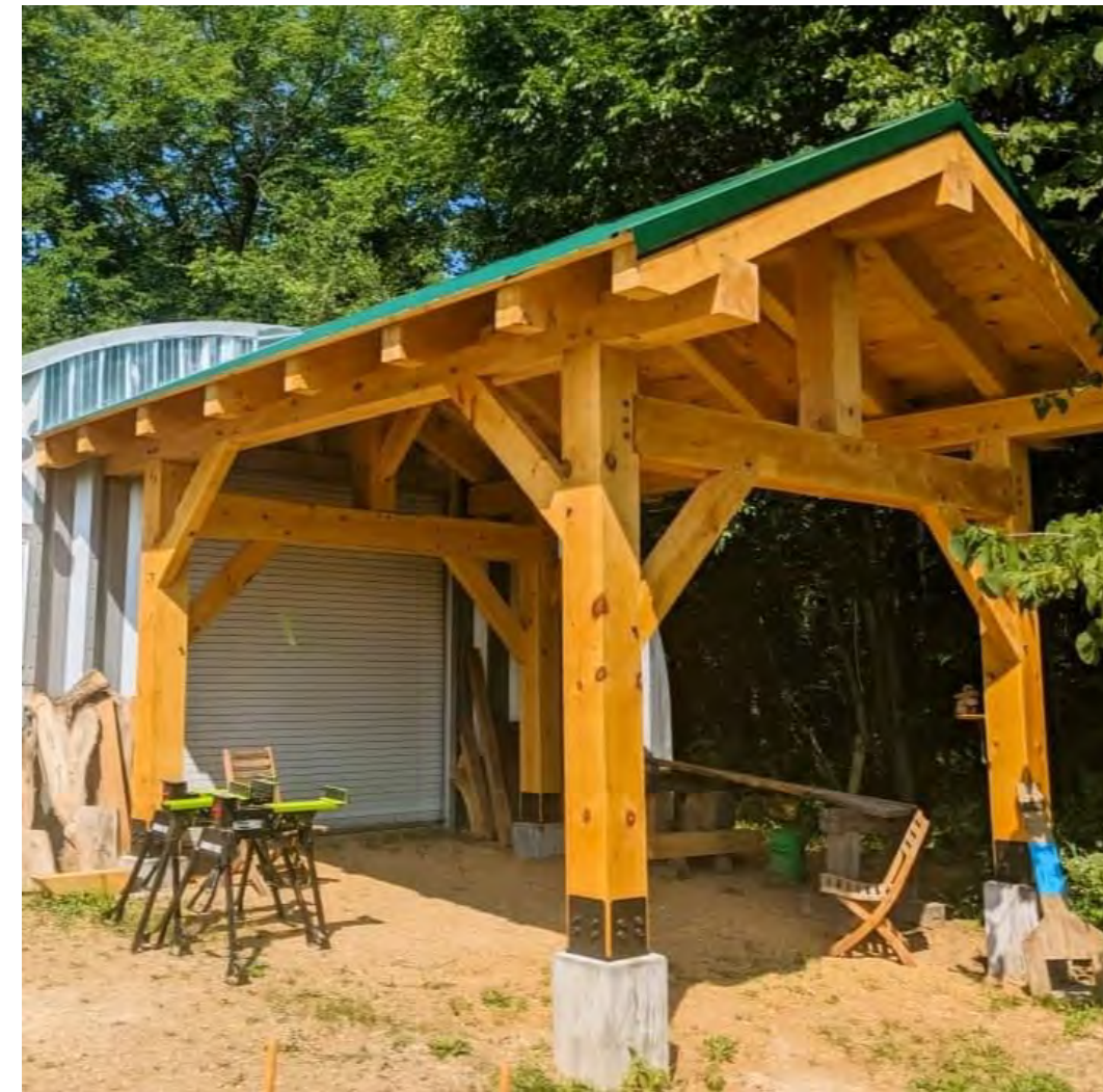
White Pine; 10" x 10" Posts, Plates, and Ridge; 10" x 12" Tie Beam; 6" x 10" Rafters ; 4" x 6" Knee Braces; 1 1/2" Tongue & Groove Decking
