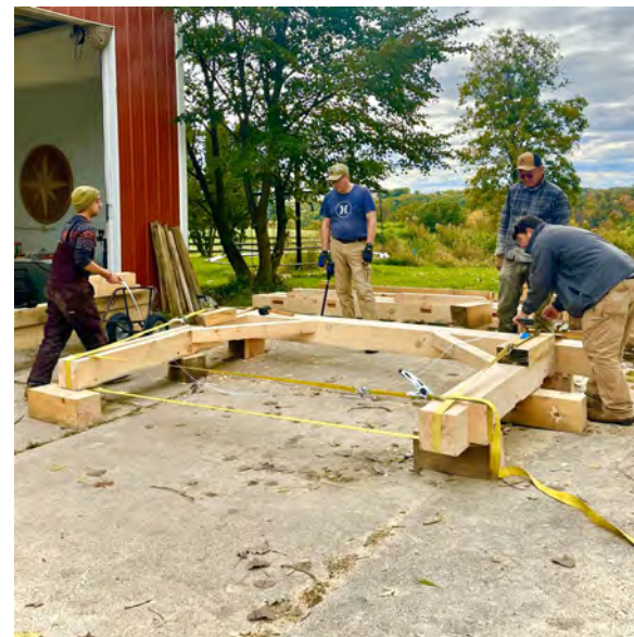
Test fitting a sauna bent
