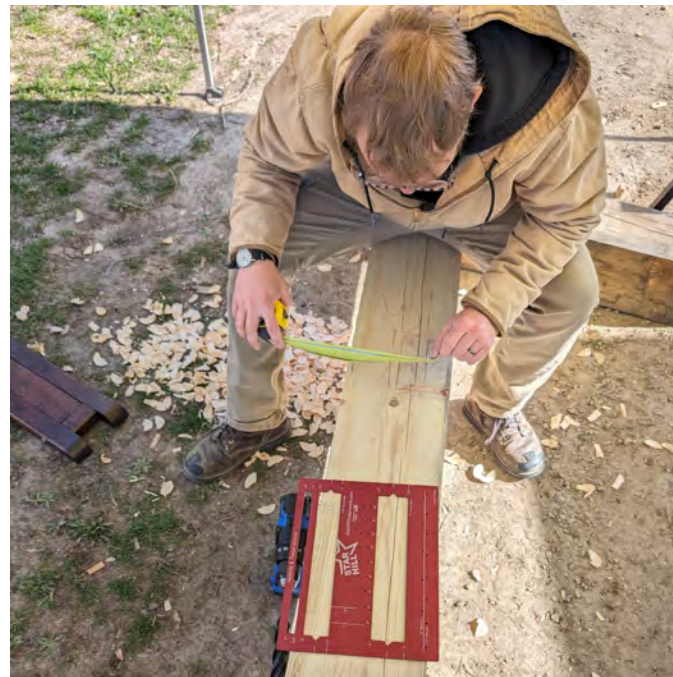
Checking timber after layout with Mortise and Tenon Master
