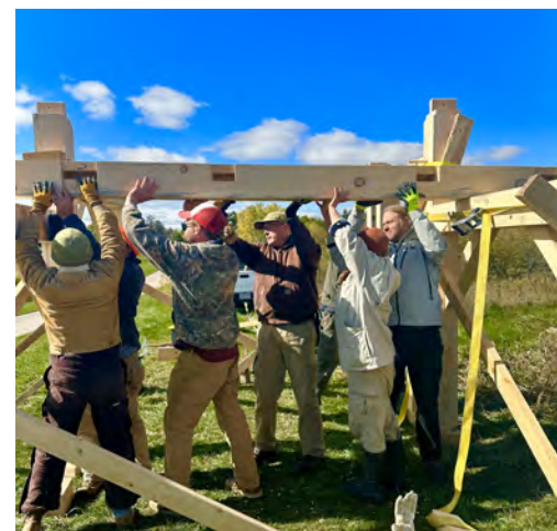
Lifting a plate by hand on raising day
