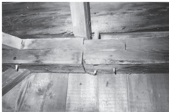
Simple bridled scarf in wall plate of five-bay barn 40 x 60 in Littleton, Massachusetts, built 1850-1870. The 2-in. tenon, 12 in. long, is secured by three pins. The builder used the same joint in the purlin plates.
