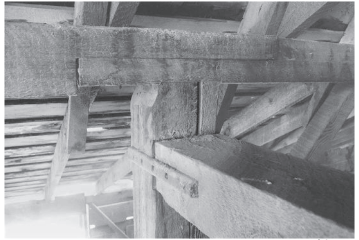
Simple halved and bolted scarf ca. 1900 near Pullman, Washington. Paul Oatman
