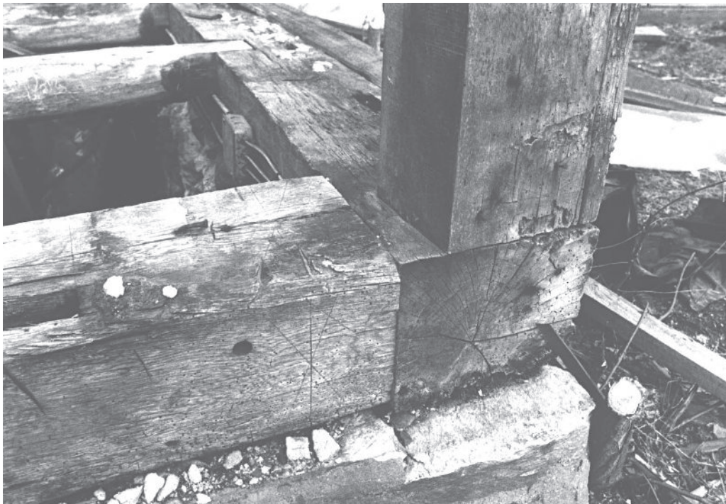
The typical blind sill corner joints on this house frame in Charlemont, Massachusetts, give little clue to their inner mortise and tenon configuration. The first joist to the rear, hewn flat only where necessary, joins the sill in a butt cog. Timber sills and girders, historically a natural part of the timber frame, have virtually disappeared from modern American work.
