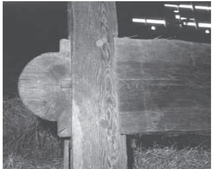
This unusual tenon profile appears on three Dutch barns in Coeymans, N.Y., likely the signature of a particular builder.
