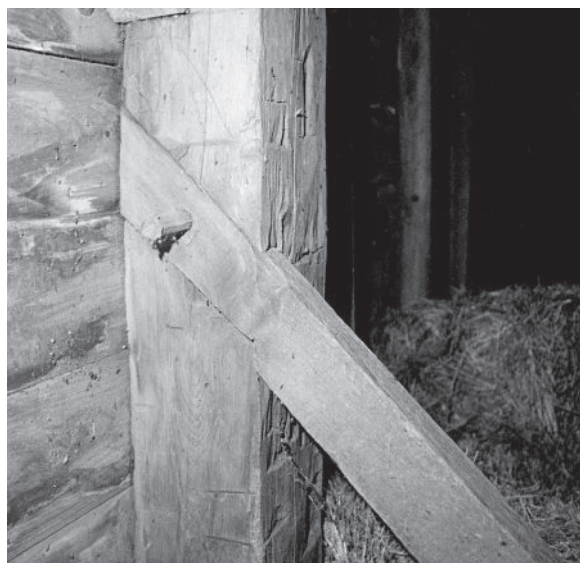
Through-lapped half-dovetails are common. The through housing removes more wood from the post than a stopped housing but can be sawn to full depth, saving considerable chiseling work. The dovetail slope is typically cut on the inner (here lower) edge of the brace. This brace runs from a post down to a tie beam in a scribe rule German barn dismantled in Alcove, N. Y., and moved to Long Island.
