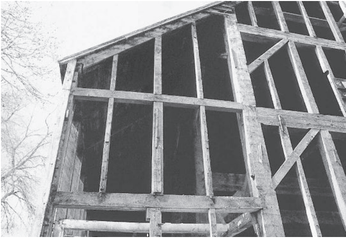
Sheathing direction determines the orientation of wall framing. This early-1800s barn (now dismantled) from Middleburg, N.Y., has studs to support wide clapboards. Note how braces take precedence over the studs.
