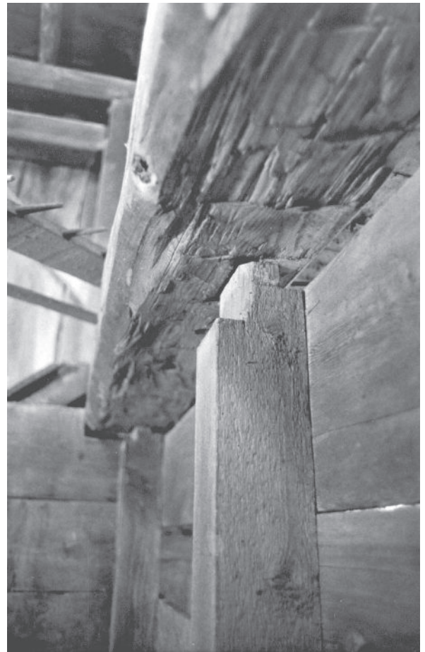
This partially withdrawn stud in a barn in Shaftsbury, Vermont, was relieved at its end to make its tenon barefaced. The relief cut was not angled as usual, and gives the appearance of a second cheek and shoulder.
