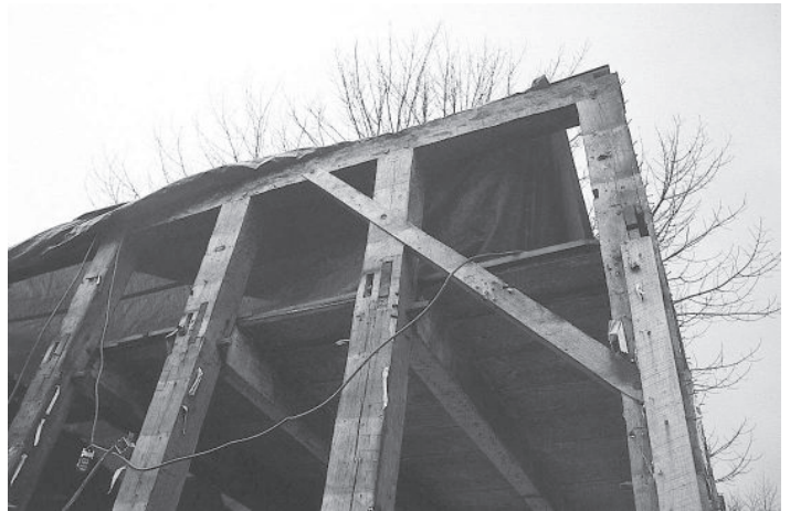
In Dutch houses with closely spaced wall posts, builders might use passing braces to achieve a long (and so more effective) brace length. In this house undergoing renovations in Alford, Massachusetts, the brace passes one post where it is lapped its full thickness and secured with a pin. Below, in lieu of normal braces, some German carpenters would angle a stud to serve as both brace and stud, as in this structure in Ephrata, Pa.
