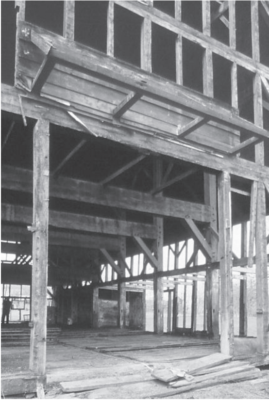
Cantilevered pentice arms run over the end anchorbeam of this Dutch barn formerly in Middleburgh, New York, and support the pentice plate with blind tenons. Rafters are butted and nailed as in Fig. 40.
