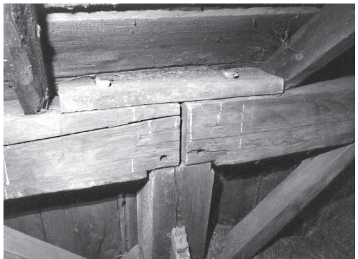
This strange arrangement in a barn in Rochester, Vermont, uses the post-top tenon as a sort of free tenon to join the plates, though pins are invisible. The builder must have realized the inherent weakness of the connection and added the fish plate on top, secured with two pins.
