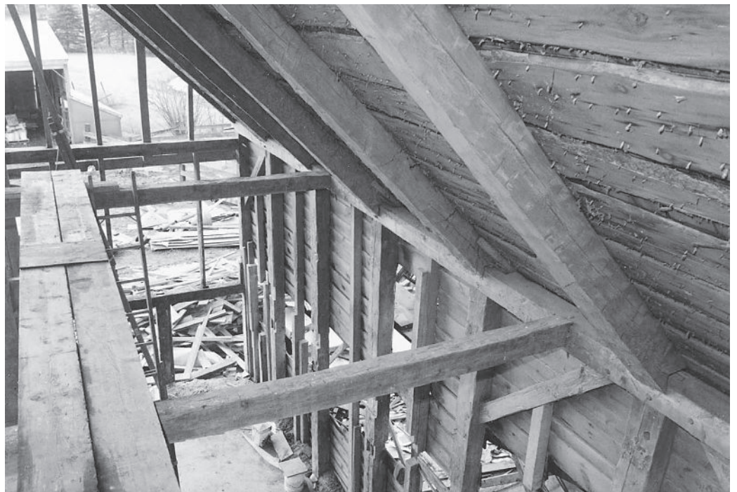
Principal rafter-common purlin roof frame over the ell of an 1840s house in Windsor, Massachusetts, now dismantled. Purlins are continuous over two bays at each end; central bay purlins are staggered on rafters for sufficient bearing at the connections. (Something went awry at the second rafter from the far end.) Instead of ridge purlins or a continuous ridge beam, purlin-runs closely flank the ridge, leaving rafter joints undisturbed at the peak.
