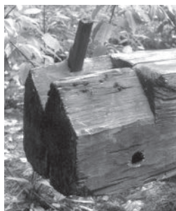
Fig. 10. Variation of the step-lap with plumb abutment. The roof plane is also elevated above the edge of the plate to increase the tail strength in this mid-19th-century carriage barn in Adams, Massachusetts.
