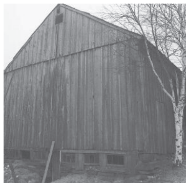
Boarding lapped at tie beam.
